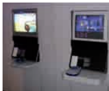
» Walls of consoles all up and running.
